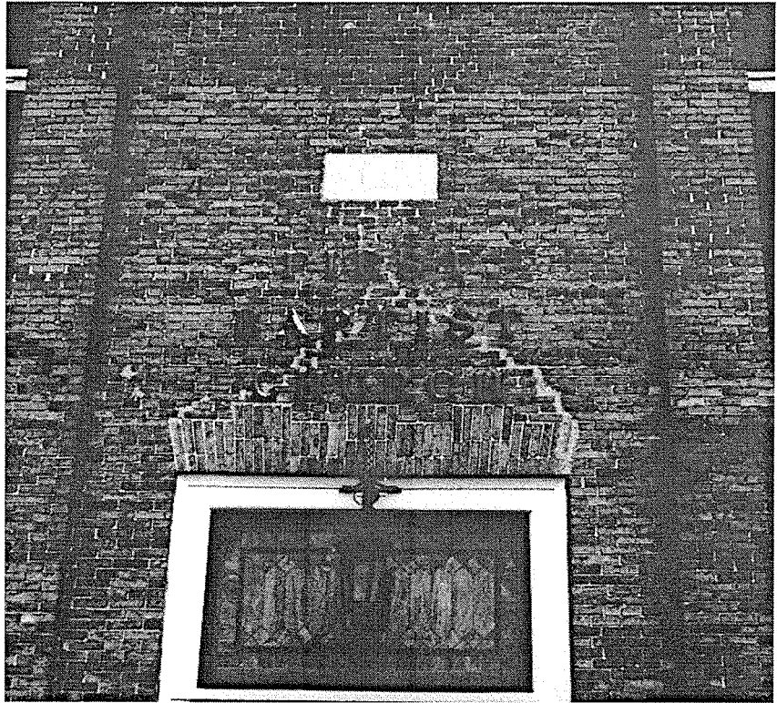
Figure 7. Cracked brick work above the main door to the First Baptist Church in Massena, corner of Main Street and East Orvis Street in Massena (Tour Stop #9). The cracks above the entrance are about 1" to 2" wide. This photo was taken in 1993.
